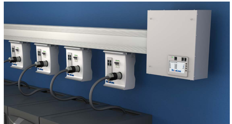
Figure 3: Busway with continuous access slot run above server racks
