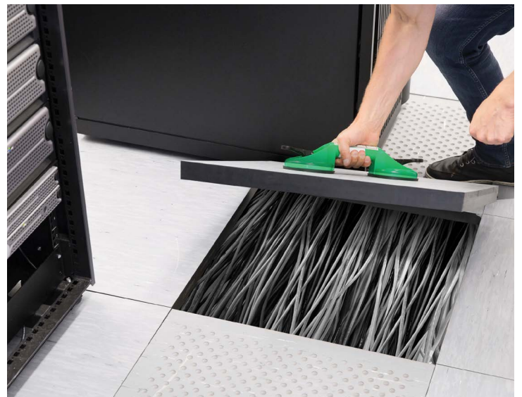
Figure 1: Traditional methods of whips and cables housed under a raised floor
