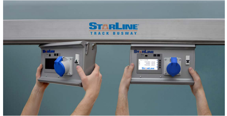
Figure 4: Example showing the ease of inserting a busway plug-in unit
