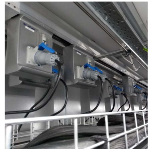
250 Amp Starline Track Busway Installed
